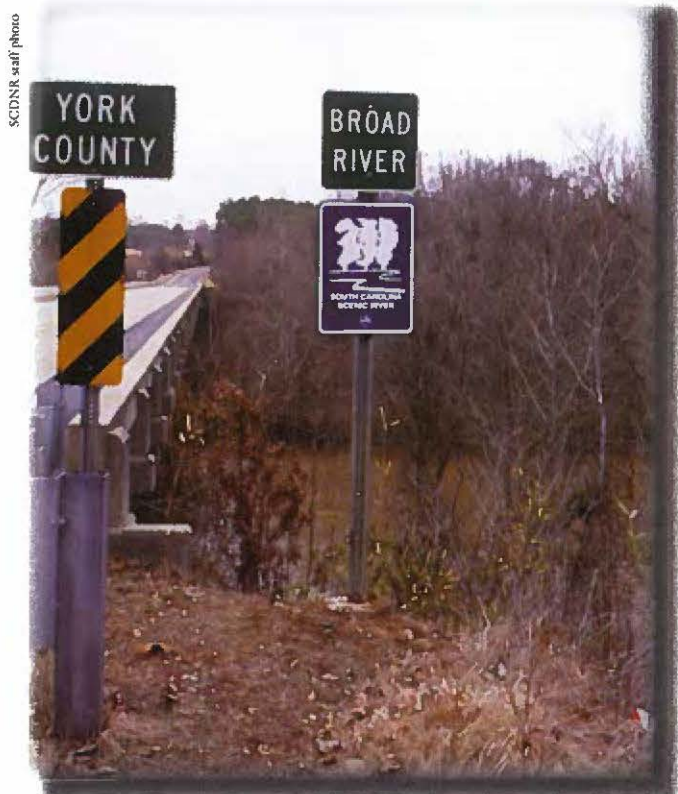
Bridge crossing at Highway 211
