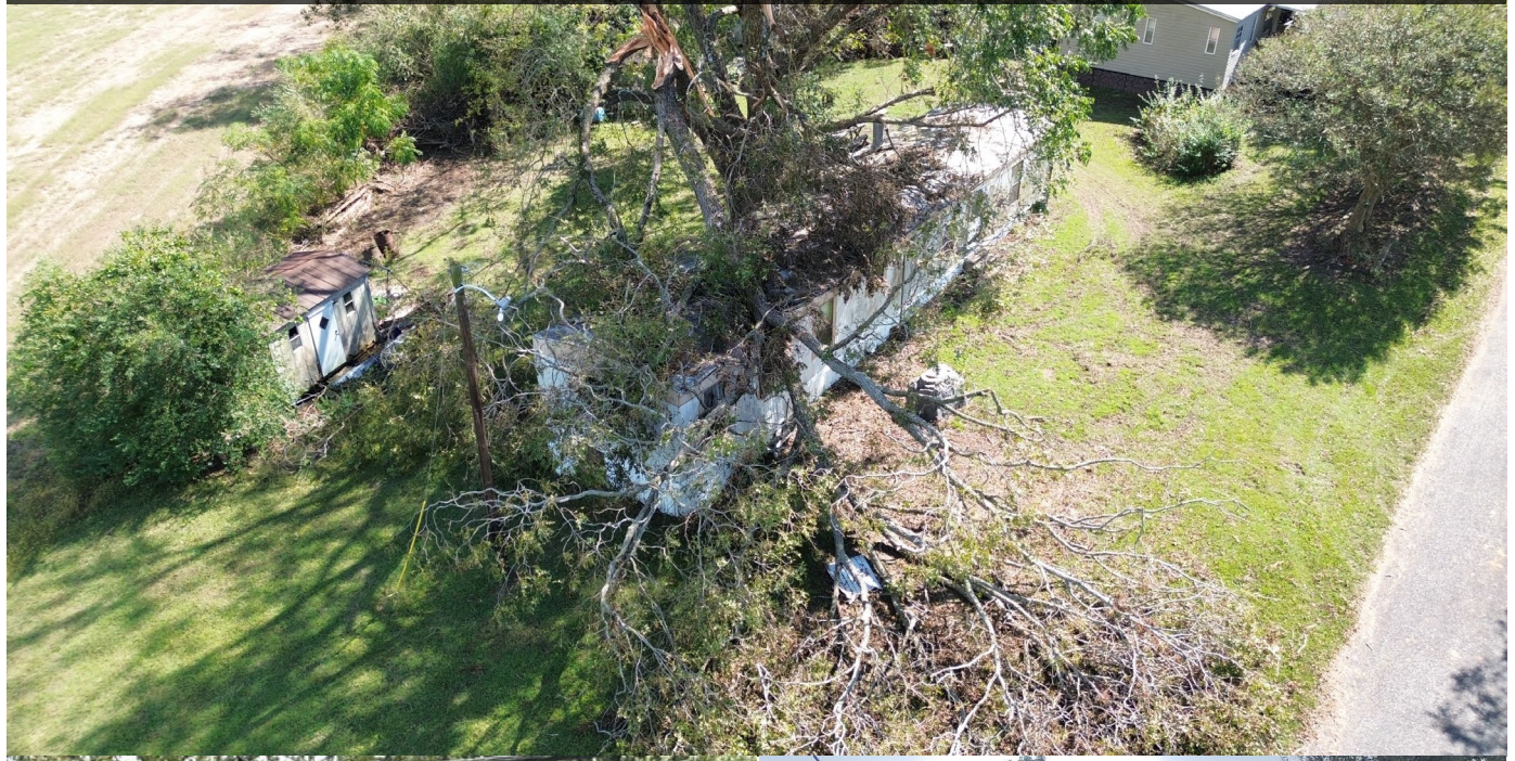
High winds downed large limbs onto this mobile home in Saluda County southeast of Saluda. SC State Guard drone photo
