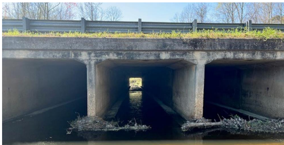
Culverts under major roads are manmade structures but do benefit bats and birds by providing roosting and nesting structure, respectively. Photo by Anna Smith, SCDNR.
