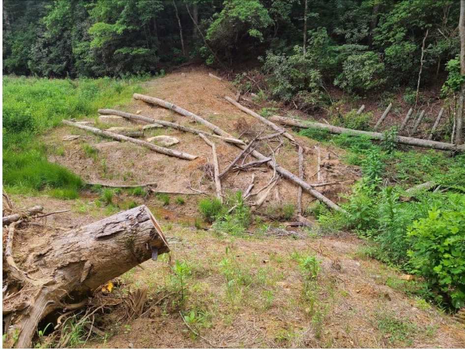
Figure 2. Photo captured by Hailey Goyette (SCDNR) of post Burrell's Pond dam removal and erosion control methods.
