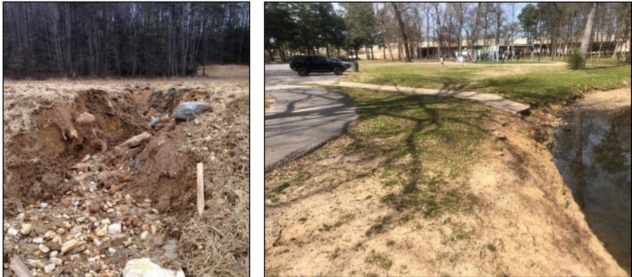
Figure 1. Examples of concentrated flow points: an agricultural ditch (left) and a storm drain (right).
