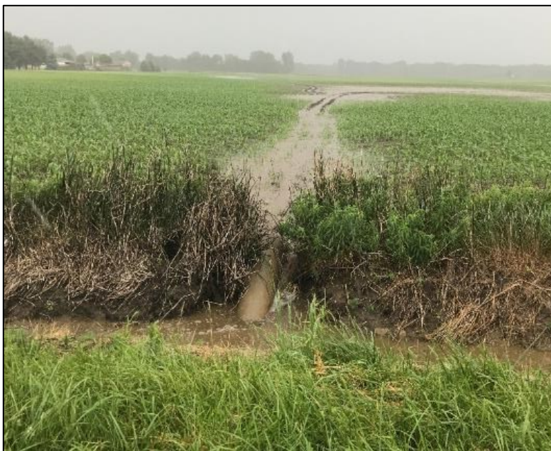
Figure 11. This agricultural drainage ditch is an example of a concentrated flow point.
