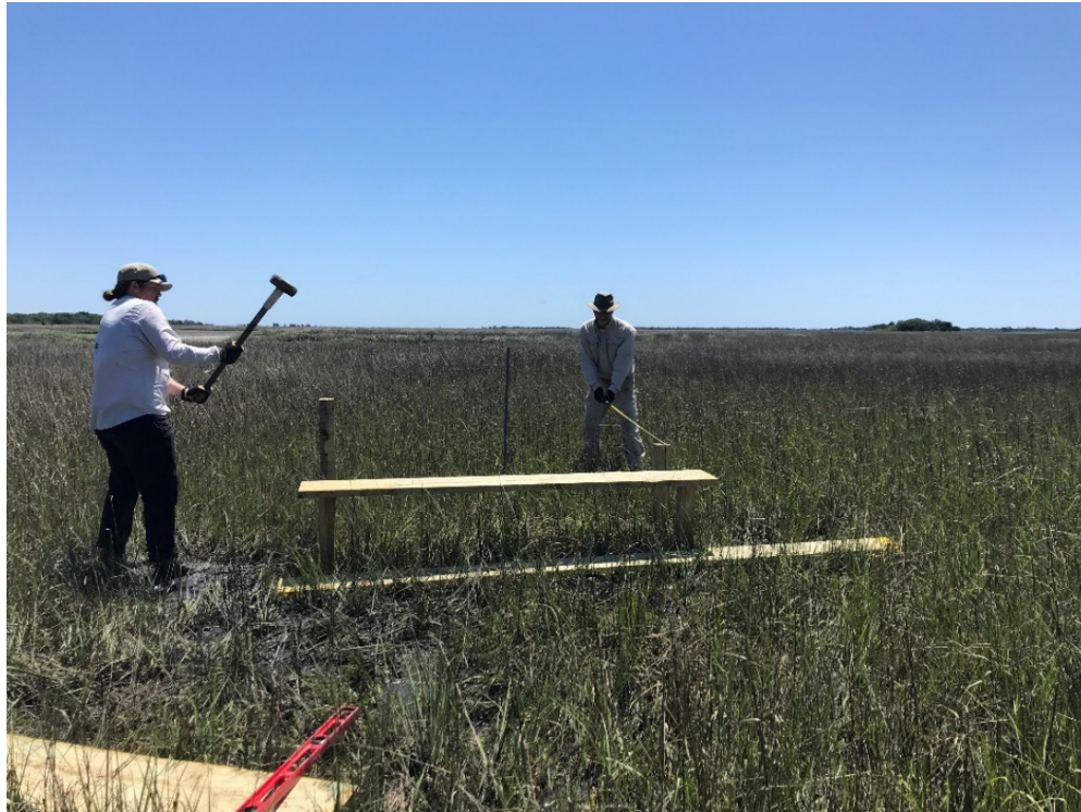
Appendix D, Figure 2. Use a sledgehammer to drive in landscaping timbers or 4x4's to create pilings (two per corner, a total of eight).
