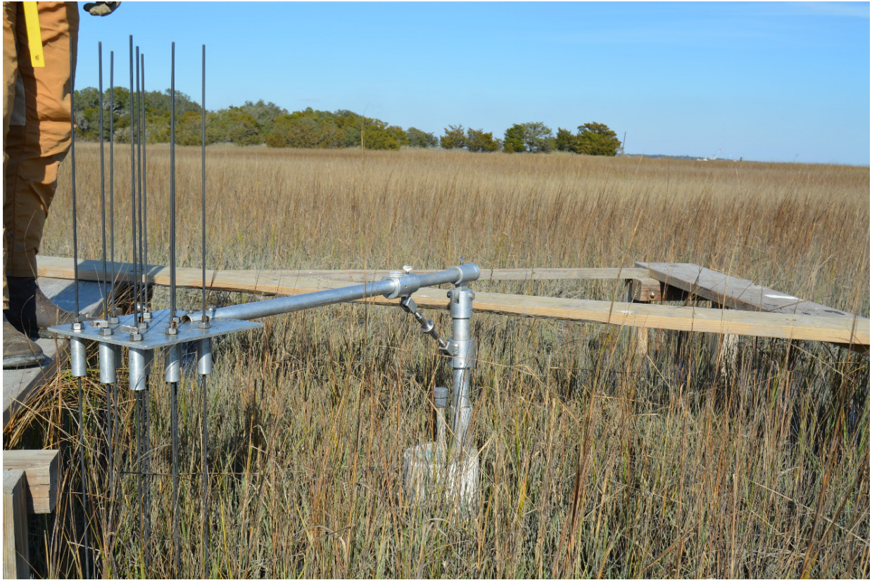
Appendix F, Figure 4. SET instrument, installed for data collection and seated directly onto insert pipe.
