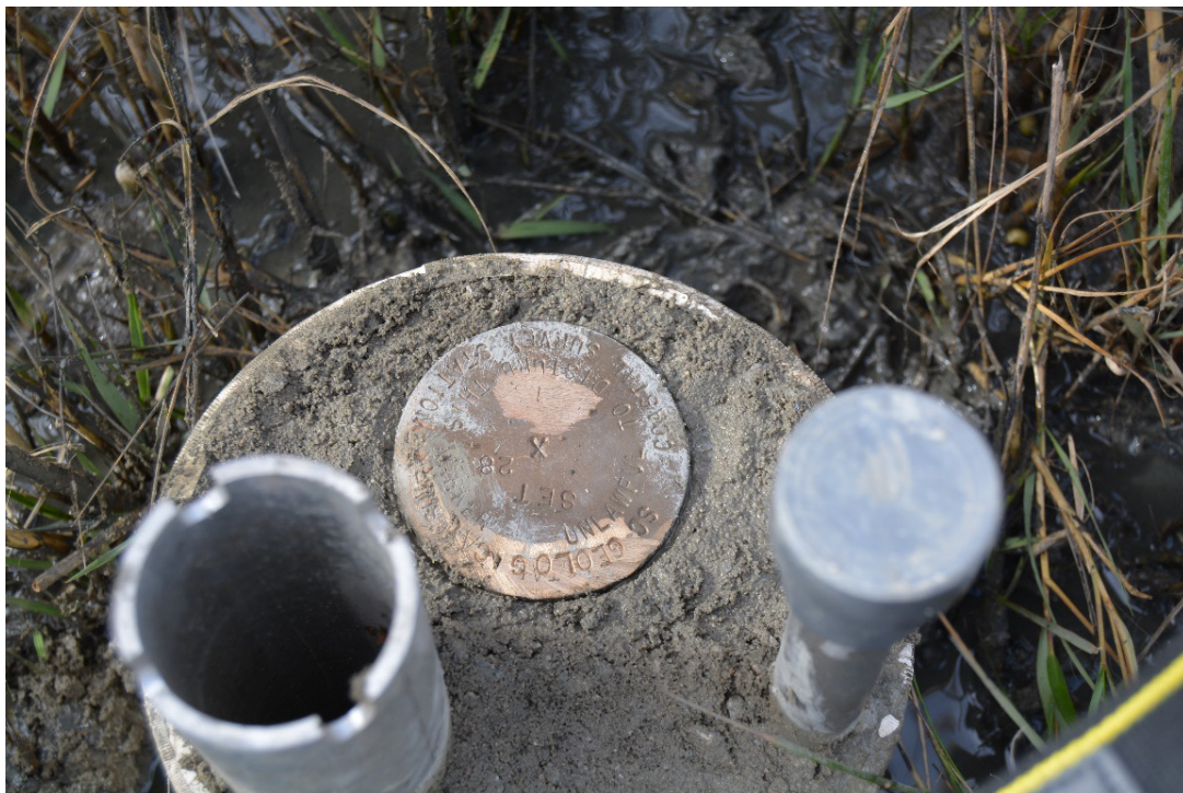
Appendix D, Figure 13. In the final stage of installation, before the concrete cures, the bronze geodetic control point disk is set into the upper surface of the concrete.
