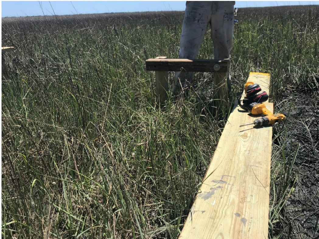
Appendix D, Figure 4. Use bolts (and washers and nuts) to attach support boards to pilings. Use a bubble level to level-in surfaces where possible.
