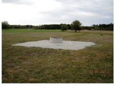
A crushed stone pad installed around the trough on top of the geotextile filter fabric provided by the Bamberg District eliminates mud and standing water.
