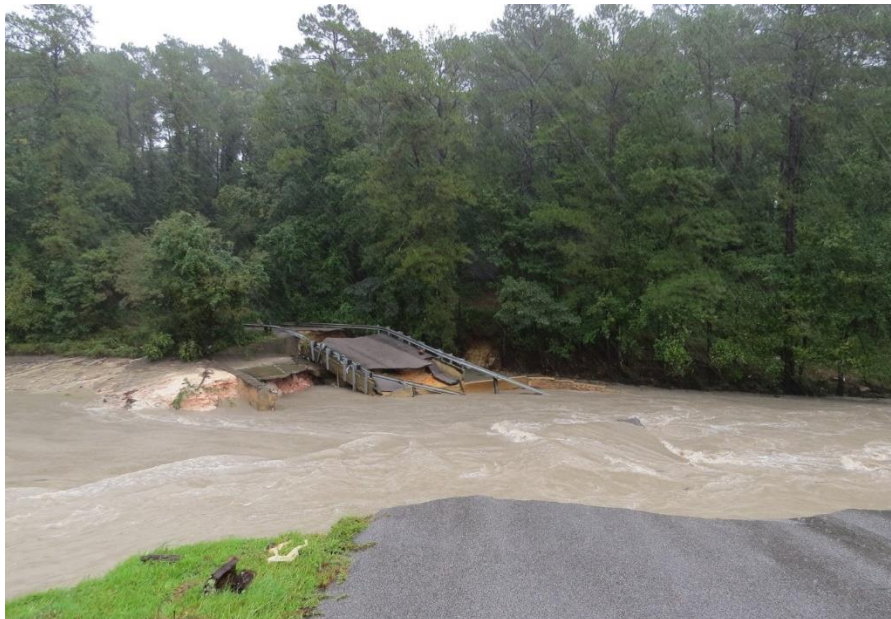
Figure 5. Cary Lake Dam Failure at Skii Lane Photo Source: Wes Tyler, SC Climatology Office
