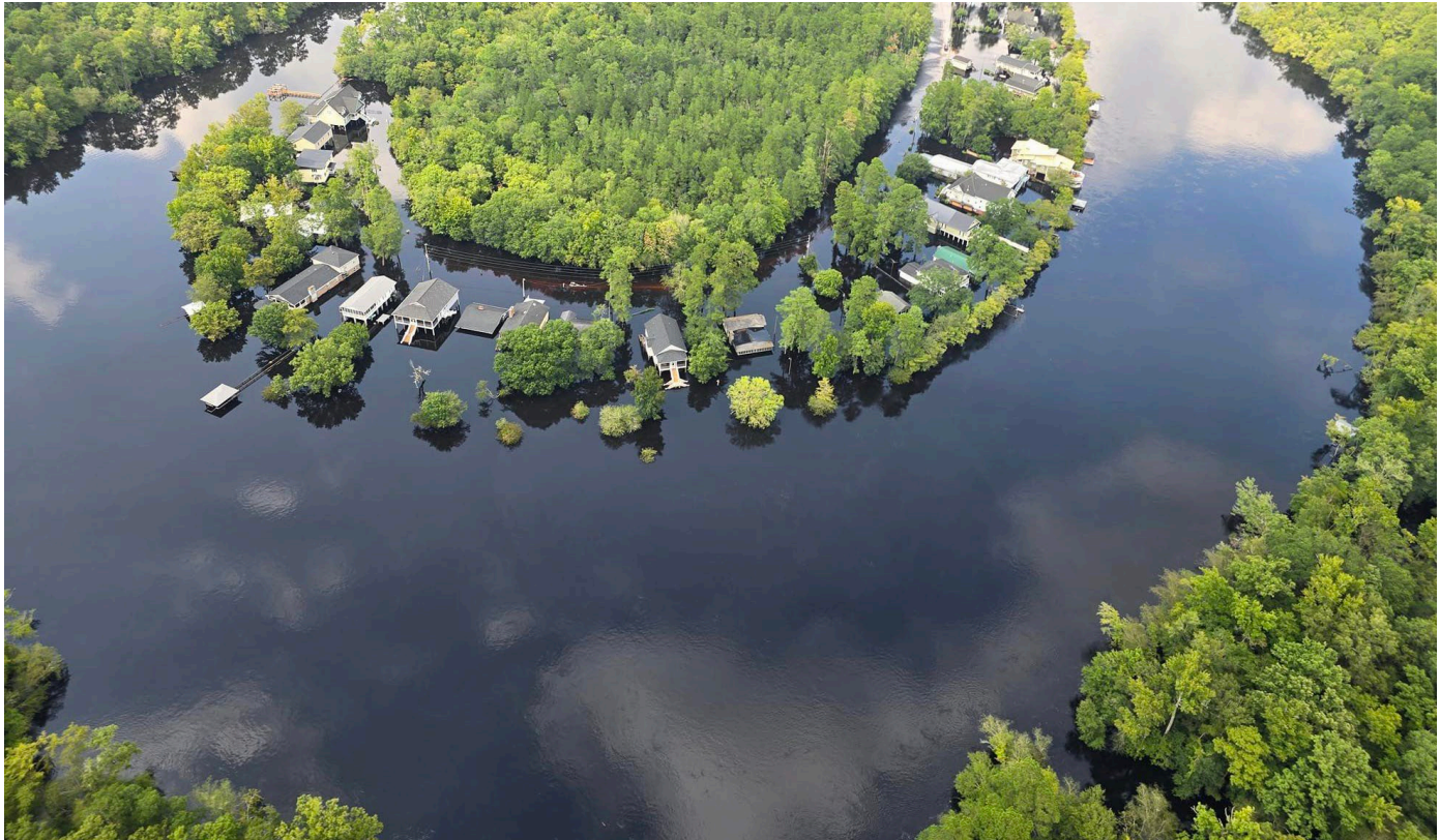
This photo of the Lumber river shows flooded homes downstream from the Nichols area.
