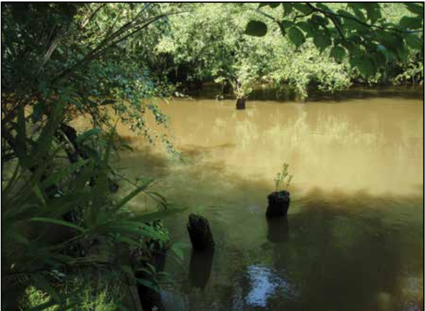
Old bridge pilings
