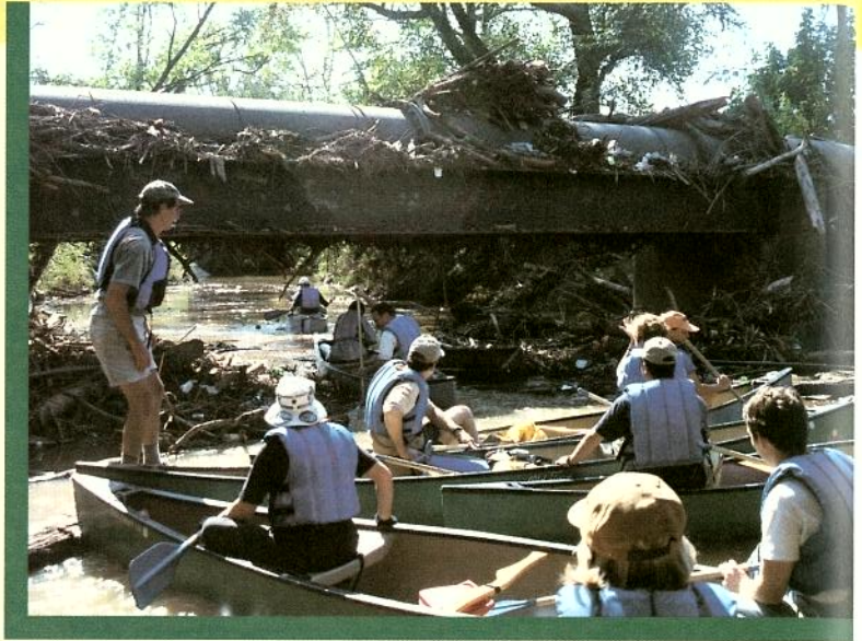
A trash and debris dam at a pipeline crossing obstructs canoeists
