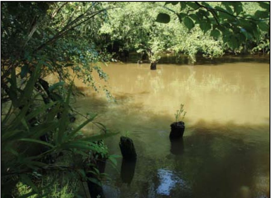
Old bridge pilings
