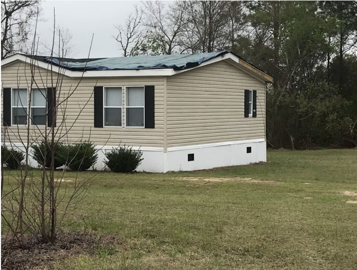
While primarily tree damage was caused by this tornado, there was some minor damage to structures, such as the shingle damage to this home.
