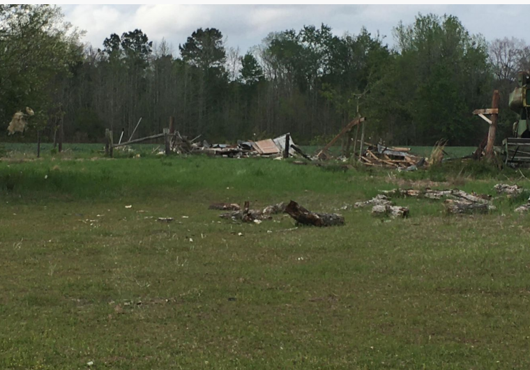
This old stick-built barn along Cramer Road in Orangeburg County was destroyed by this tornado.
