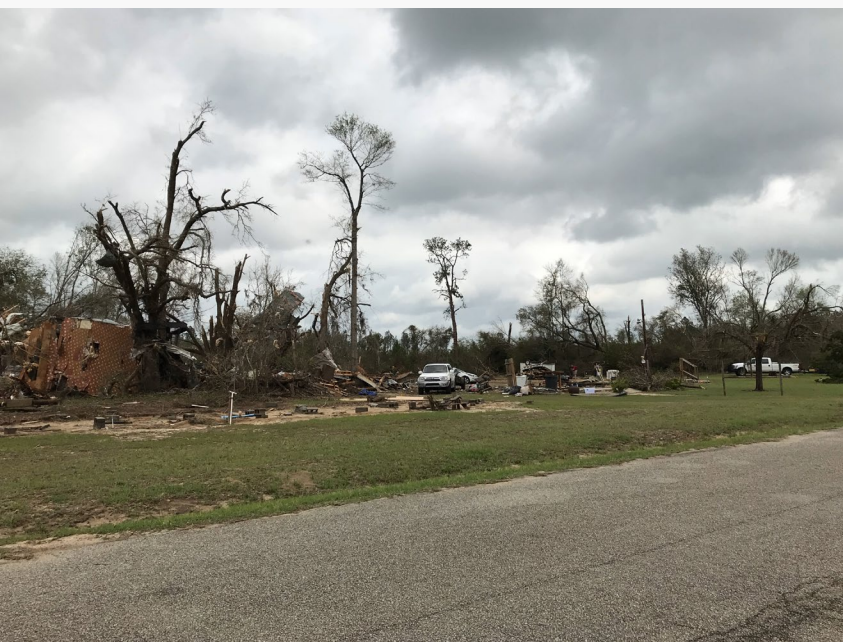
One of a few mobile homes that were demolished by this tornado southwest of Allendale. Also, the mobile home's undercarriage was lifted and moved about 30 feet. Significant tree damage is also evident.
