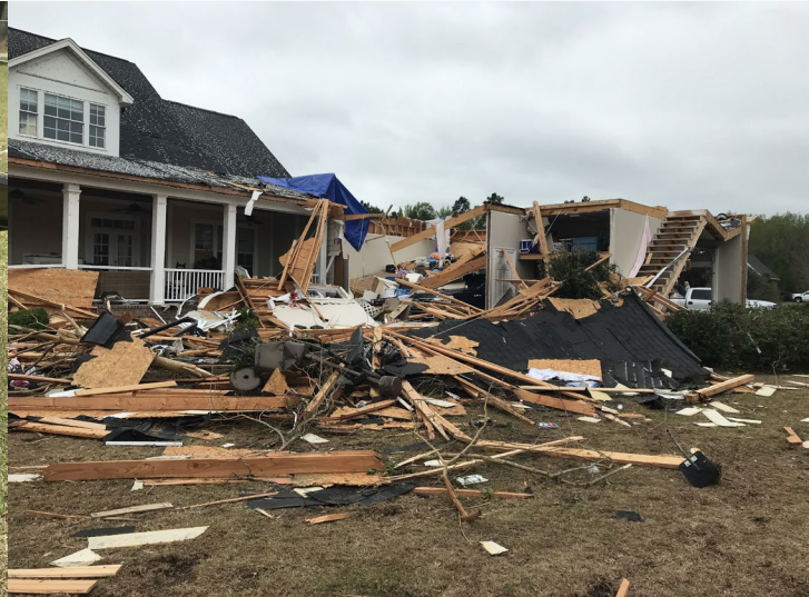
A photo of significant damage to a residence on Gossett Court north of Manning. Hurricane clips on this home's roof likely prevented even worse damage.
