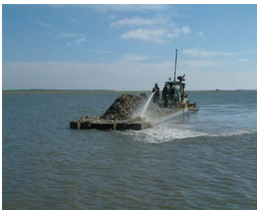
Figures 2. and 3. Quarantined Gulf Coast oyster shells are floated off a contractor's barge (left) onto a previously designated restoration area using high pressure water cannon at high tide. Results of intertidal planting after PVC poles have been removed are shown (right).
