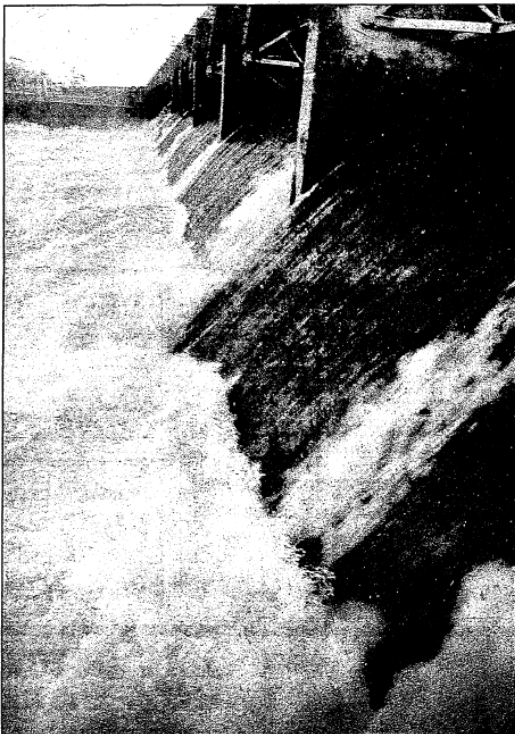
Water pours through the floodgates of the Santee Dam at a rate of almost 300,000 gallons per second Monday as Santee Cooper officials open the gates to eight feet to lessen the pressure on the dam from water flowing into Lake Marion. The water comes from rivers swollen from rain spawned by the remains of Tropical Storm Marco. See story, Page 3-B.
