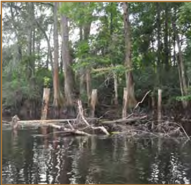
Old bridge pilings
